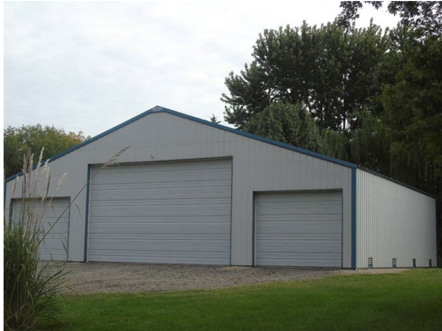
Figure 3: Agricultural Structure for Equipment and Storage, with Flood Openings (Source: Steve Samuelson, Kansas NFIP Coordinator)
