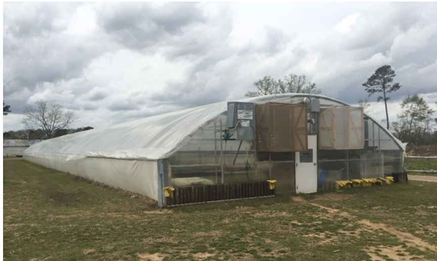
Figure 14: Greenhouse with Flexible Sides and Removable “Roof”
