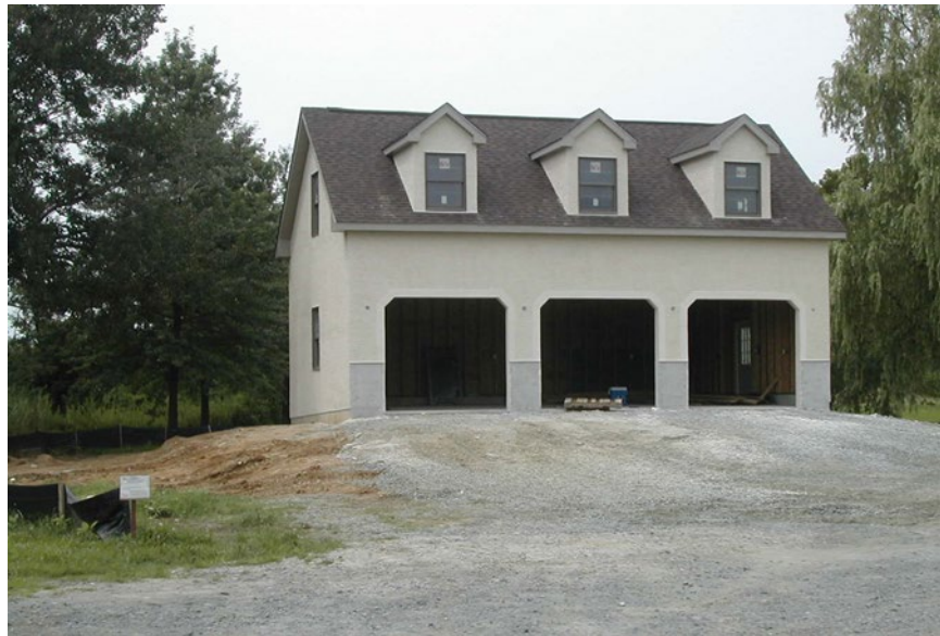
Figure 22: Three-Car Garage Elevated on Fill
