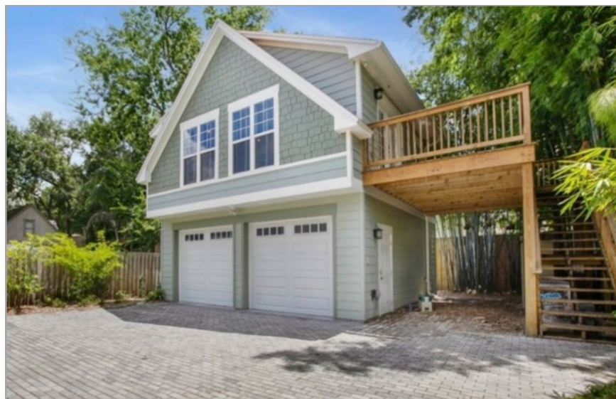
Figure 17: Elevated Accessory Residential Structure, with Enclosure
