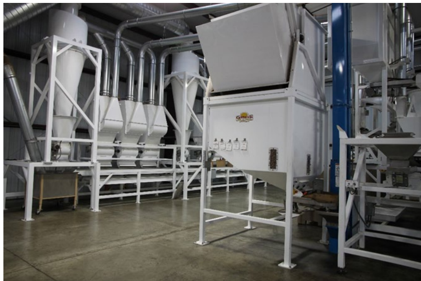
Figure 11: Structure Used for Processing Nuts
