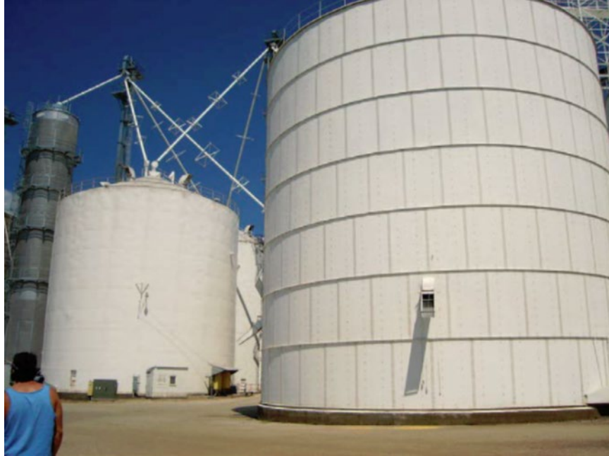
Figure 5: Welded-Seam Silo (Left) may be Watertight; Bolted-Plate Silo (Right) is not Watertight
