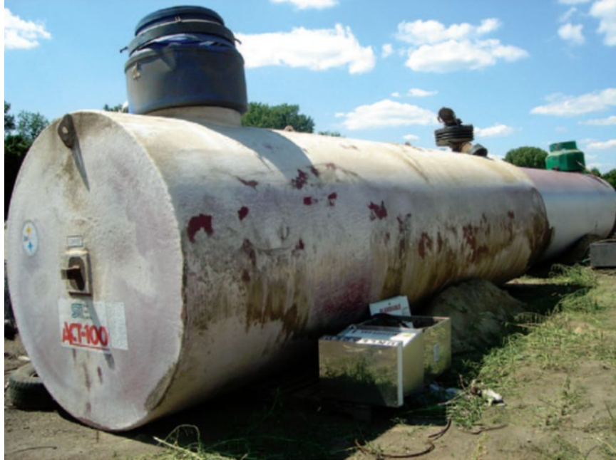
Figure 6: Buoyancy Forces Dislodged Two 10,000-Gallon Underground Fuel Tanks
