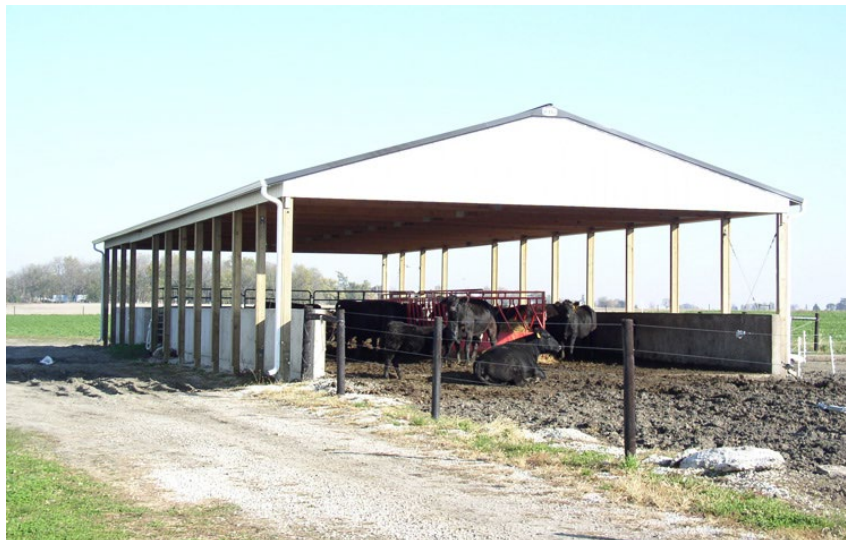
Figure 13: Pole Barn Without Walls (Source: USDA Agricultural Research Service, 2011)
