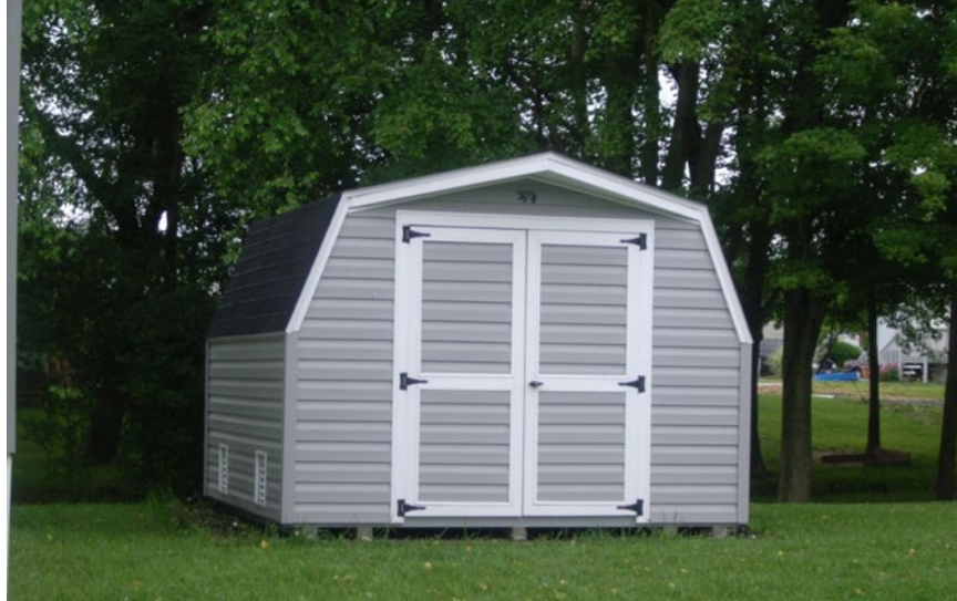
Figure 16: Storage Shed, with Flood Openings (Source: Kevin Wagner, Maryland Department of the Environment)
